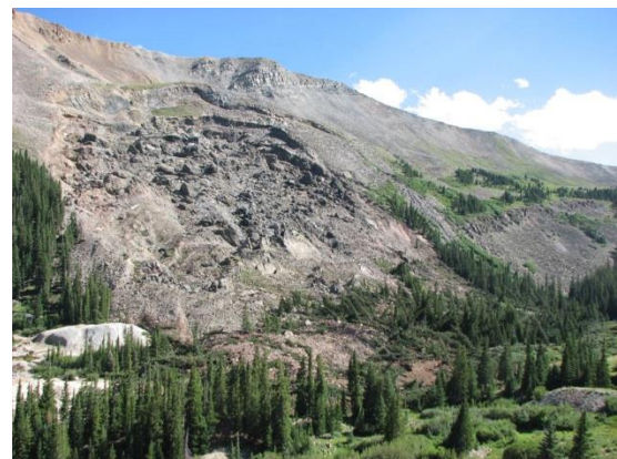
2011 landslide along West Mosquito Creek in Park County, Colorado.
