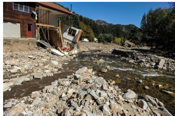
Aftermath of 2013 flood in Jamestown, CO.
