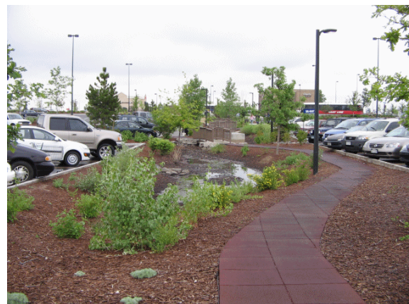
Example of LID (bioswale) in large commercial parking area in Aurora, CO.
